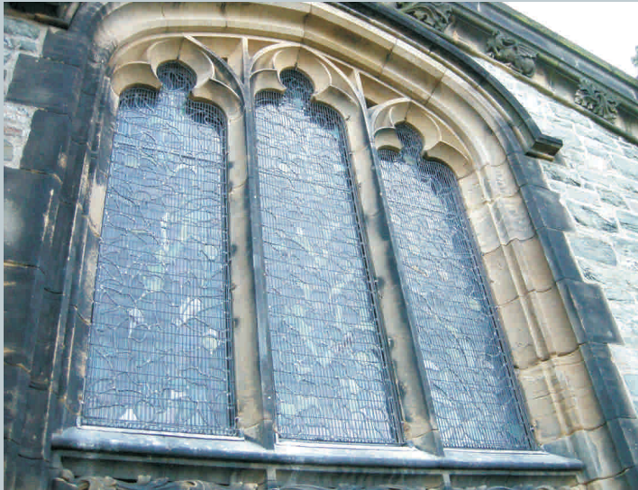
The William Morris Tree of Life Window, St. Cybi's Church Holyhead Stainless Steel, Powder-Coated Guards were Installed on Completion
